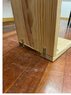
(e) External connection between pillar and base
