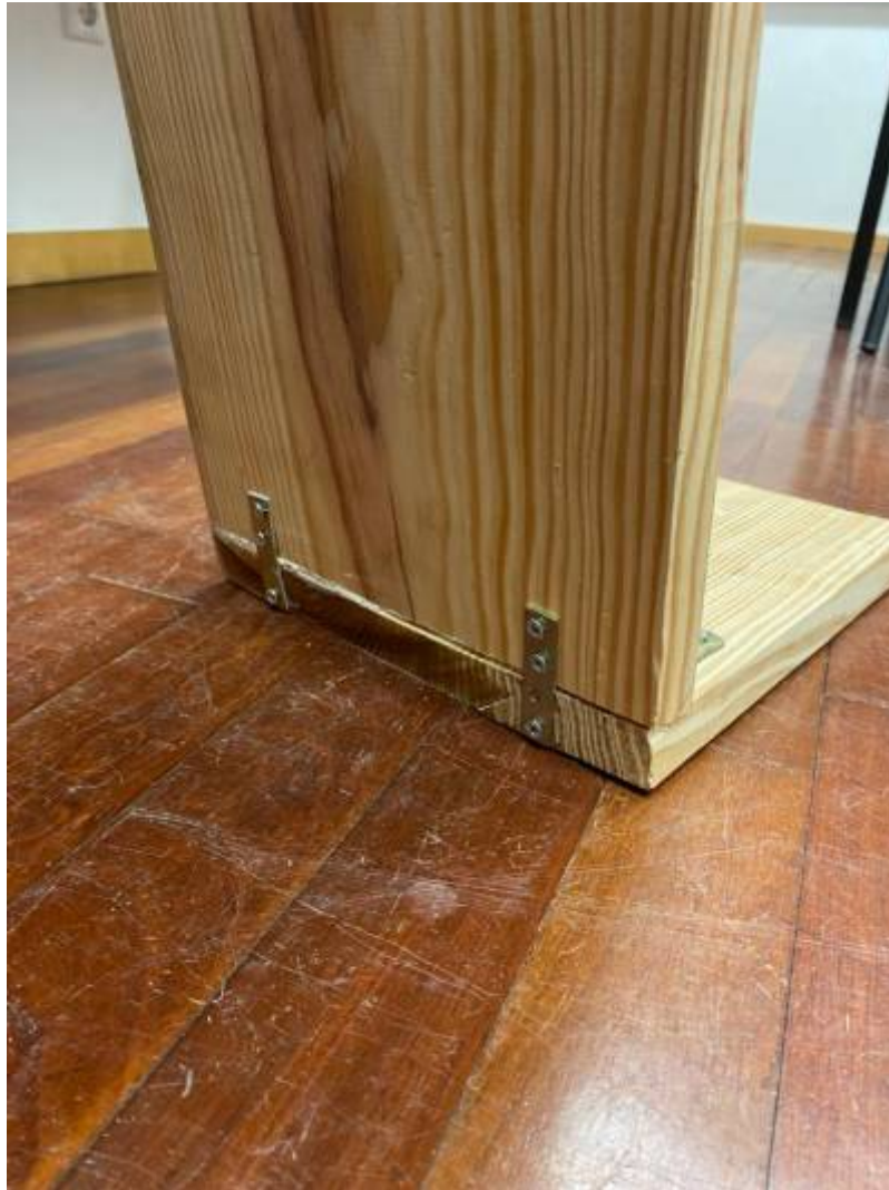
Figure 55: External connection between pillar and base
