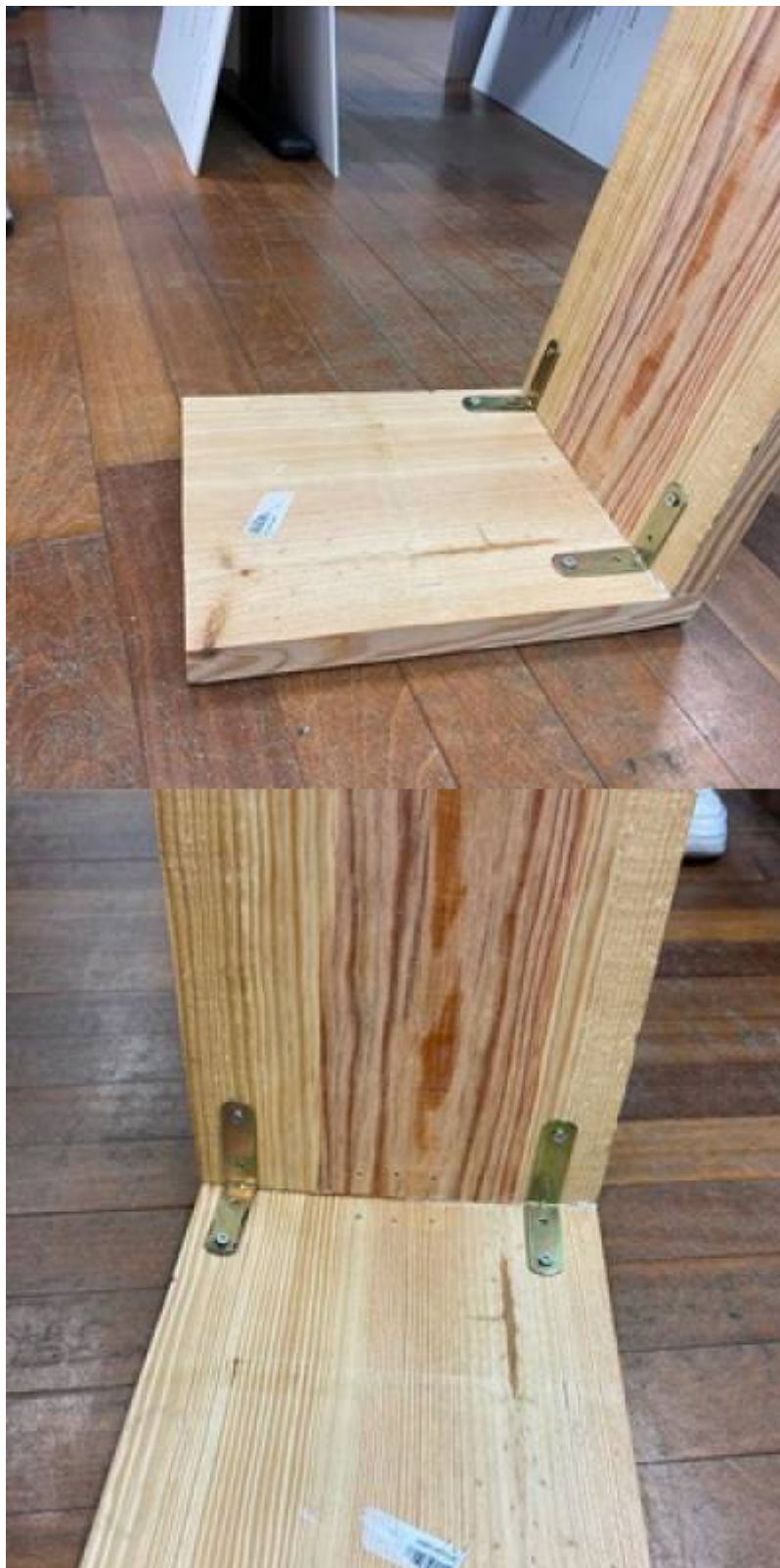
Figure 54: Internal connection between pillar and base
