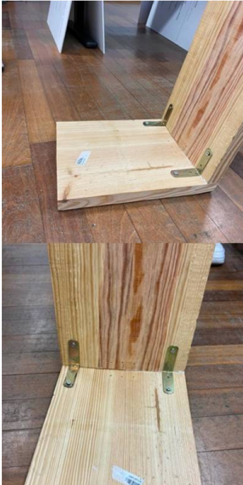
Figure 55: Internal connection between pillar and base
