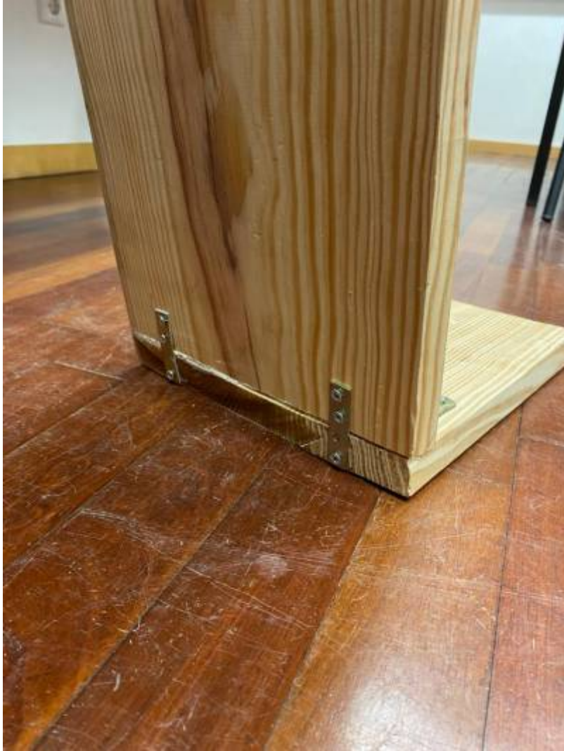
Figure 56: External connection between pillar and base
