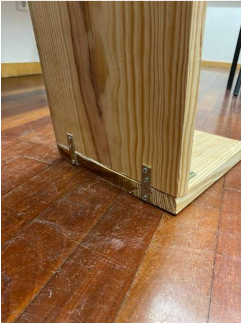
Figure 56: External connection between pillar and base
