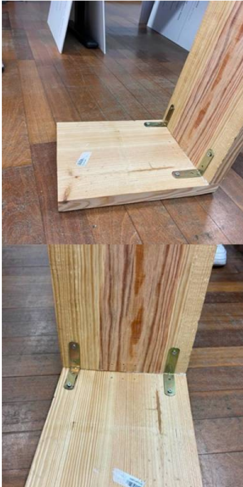
Figure 55: Internal connection between pillar and base
